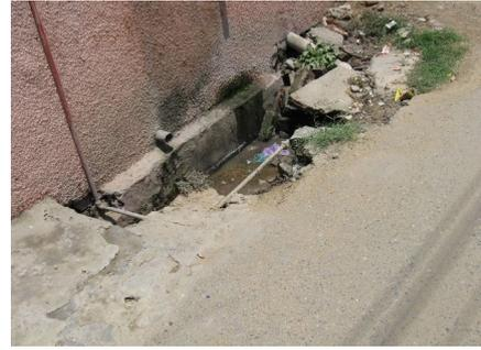
**Fig no.36: Open drain along road****5.1.3 STORM WATER DRAINAGE**
